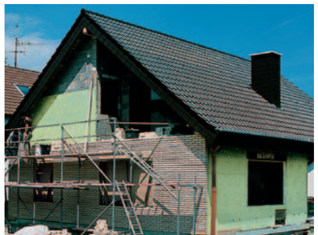
Fig. 39: Cavity wall insulation with Styrodur C.
