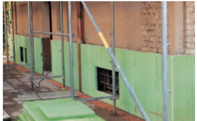
Fig. 17: Subsequent base insulation with Styrodur 2800 C.
