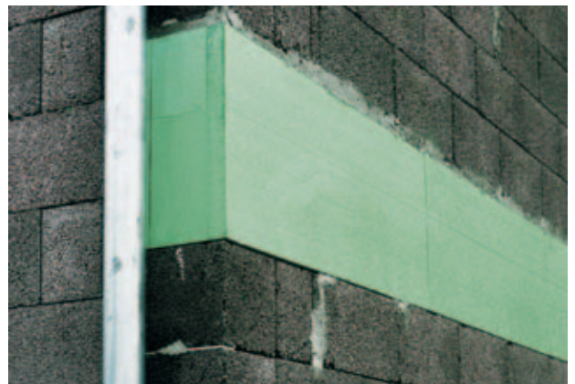
Fig. 2: Insulation with Styrodur® 2800 C at the ceiling edge.
