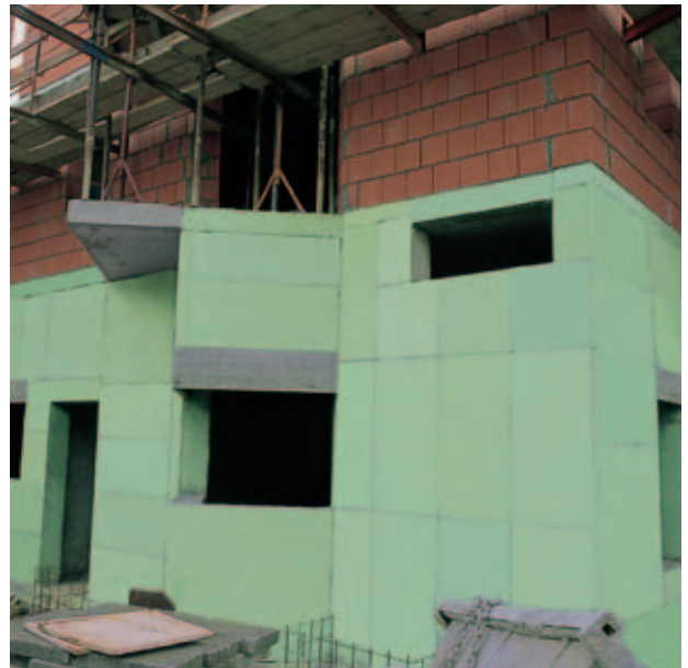
Fig. 25: Large-sized ground floor insulation with Styrodur C boards.
