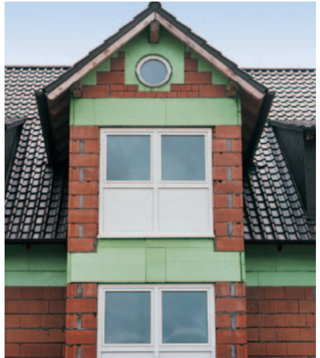
Fig. 1: Insulation of cold bridges in concrete units: – verge – ridge support – ring beam – lintel – edge of ceiling
