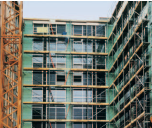
Fig. 7: Cold bridge insulation with Styrodur® 2800 C.
