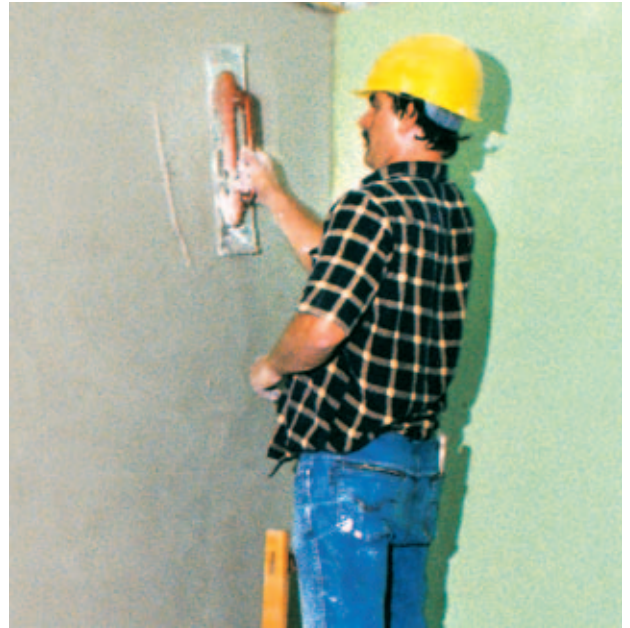
Fig. 34: Applying the second layer of plaster (5 mm), using the wet-on-wet method.
