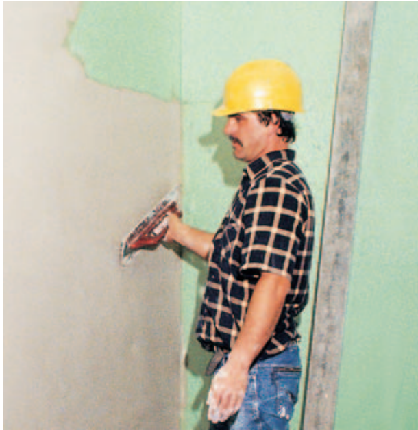
Fig. 32: Applying the first layer of bonding plaster (10 mm).
