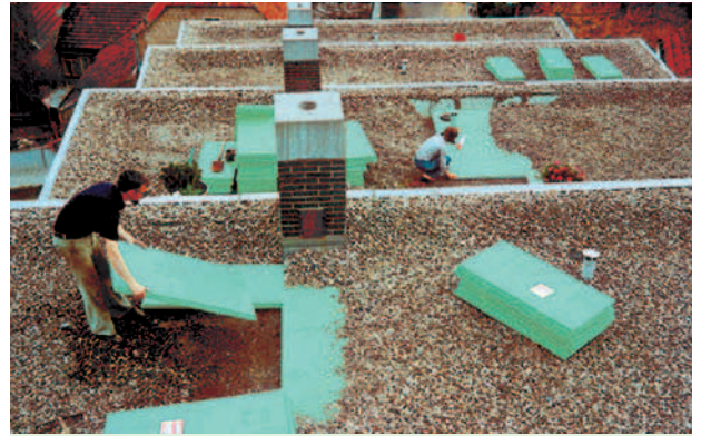
Fig. 1: Due to its compressive strength, low water absorption, and low thermal conductivity, Styrodur® C is perfectly suited for inverted roof structures, such as plus roofs for flat roof renovations.
