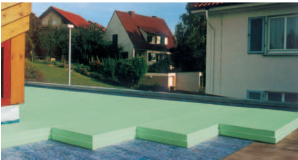
Fig. 26: Installation of Styrodur® C boards under an extensive green roof.
