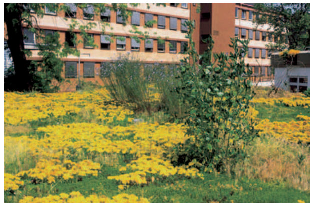
Fig. 24: Vibrant urban landscapes can be achieved with a green roof on Styrodur® C.
