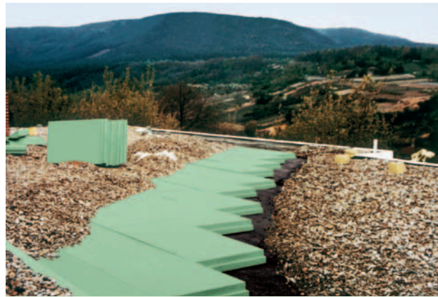
Fig. 17: Renovated inverted roof in the form of a plus roof.
