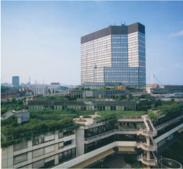
Fig. 28: Intensive green inverted roof.
