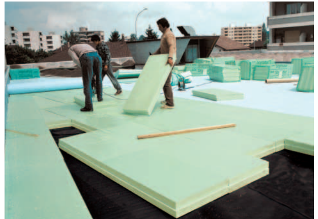
Fig. 13: Installation of Styrodur® C on a duo roof.
