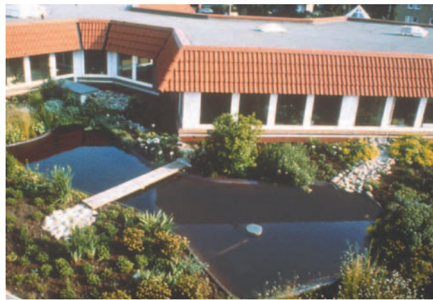
Fig. 23: Vegetated walkable roof terrace with pond irrigation system on an inverted roof design with full gravel drainage layer.
