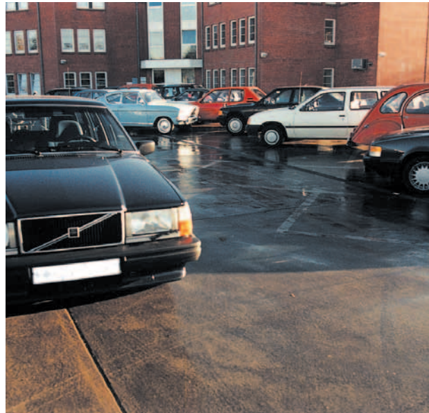
Fig. 51: Parking roof with in-situ concrete driving surface.
