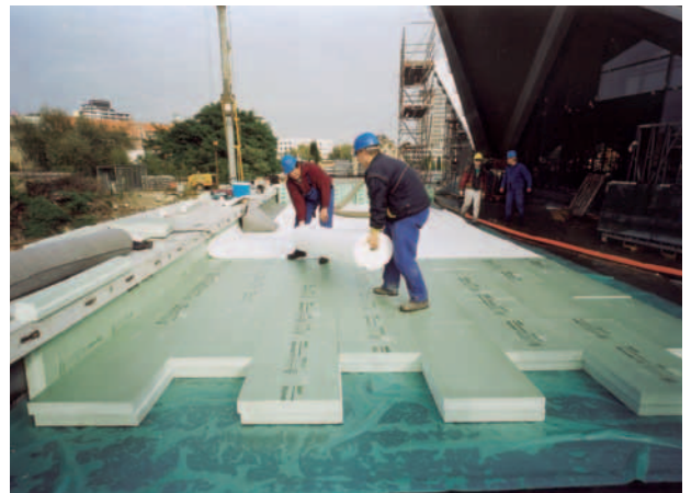
Fig. 15: Installation of Styrodur C on top of the roof waterproofing.
