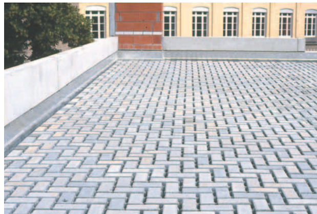
Fig. 49: Concrete pavement on Styrodur® C boards.
