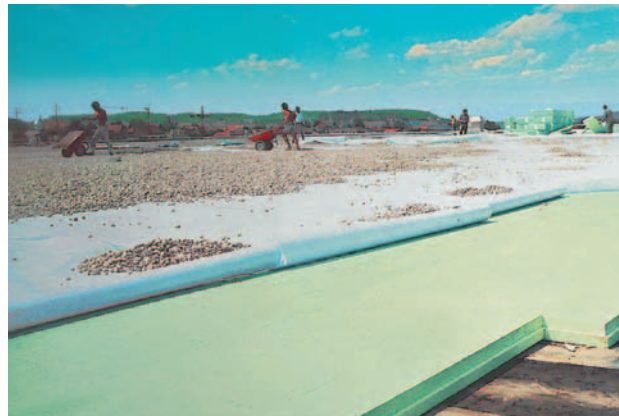
Fig. 9: Inverted roof with separation layer and gravel.
