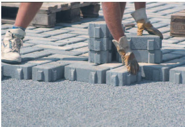
Fig. 48: Composite stone pavement with grass joints for a parking roof on top of a gymnasium.
