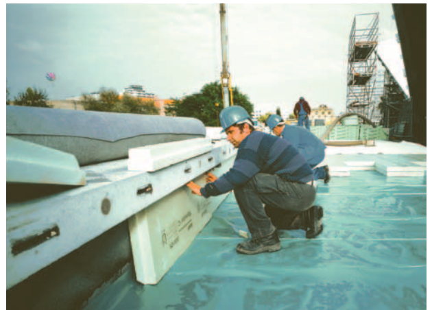
Fig. 14: Parapet insulation with Styrodur C.
