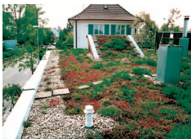
Fig. 36: Gravel shoulder along the roof edge and roof penetrations.
