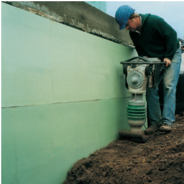
Fig. 28: Layered backfilling of the excavation pit and mechanical compacting.
