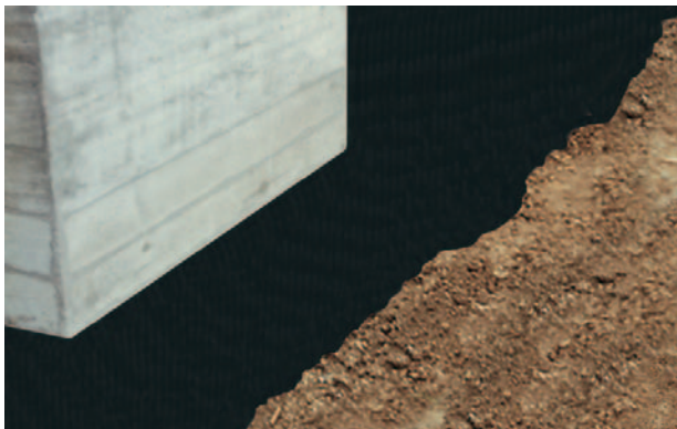
Fig. 15: Waterproofing the basement walls against pressing water.
