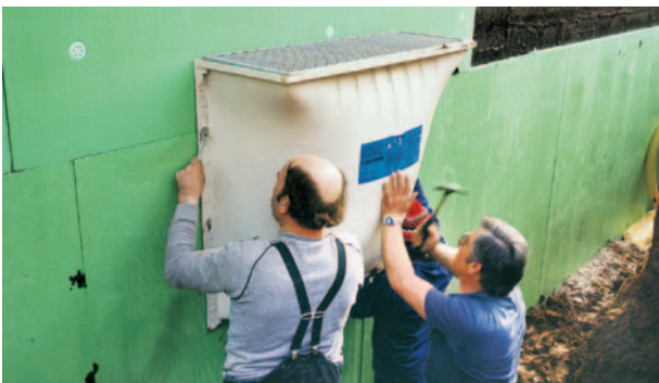
Fig. 22: Lightwell assembly with perimeter insulation.
