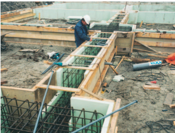
Fig. 25: Formwork with Styrodur® C.
