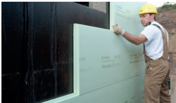
Fig. 4: Styrodur® C boards provide perimeter insulation without thermal bridges.
