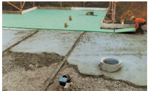
Abb. 6: Blinding layer of lean concrete for the installation of floor insulation
