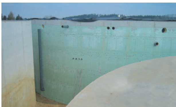
Fig. 1: Styrodur® C thermal insulation on a reinforced concrete fermenter wall.
